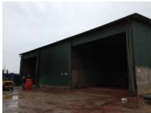
Blasting & Painting Area
