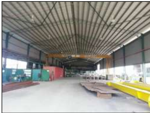
Open Fabrication Area
